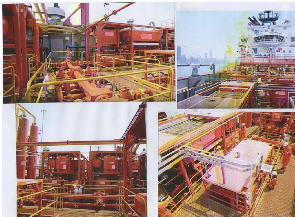
Figure (3) Photos of Typical HCl Acid Processing Equipment on board a ship classed by Lloyd's Register [Courtesy of OML (Overseas Marine Logistics L.L.C.)]
